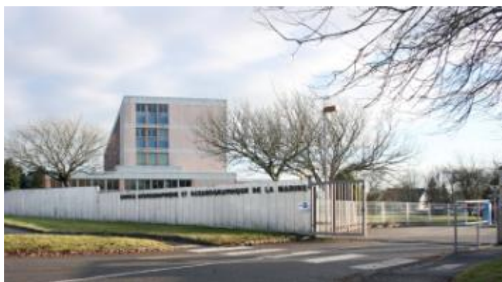
Fig. 1. SHOM facilities in Brest
